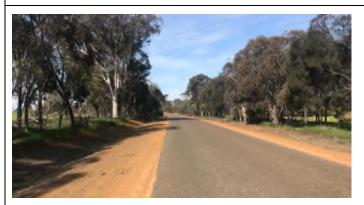
Road seal edge and shoulders are in good condition. Minimal signs of drop off or edge damage.
