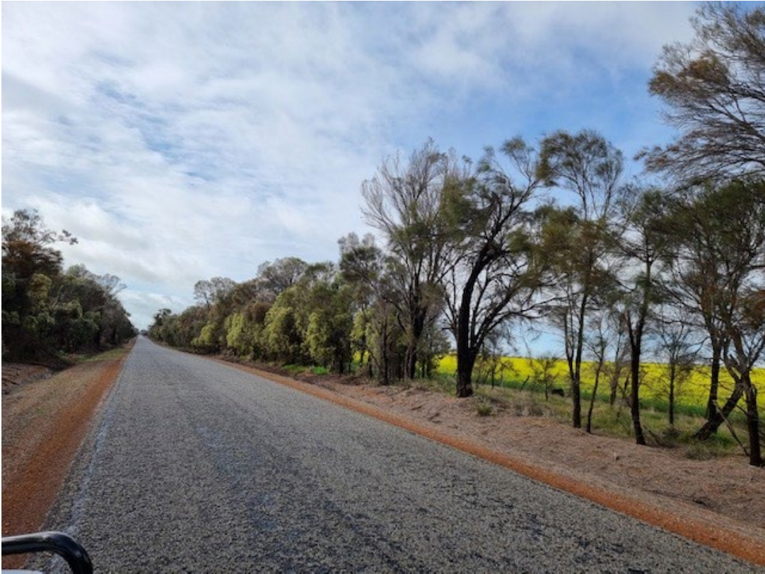
Figure Two – Facing South on Shenton Road
