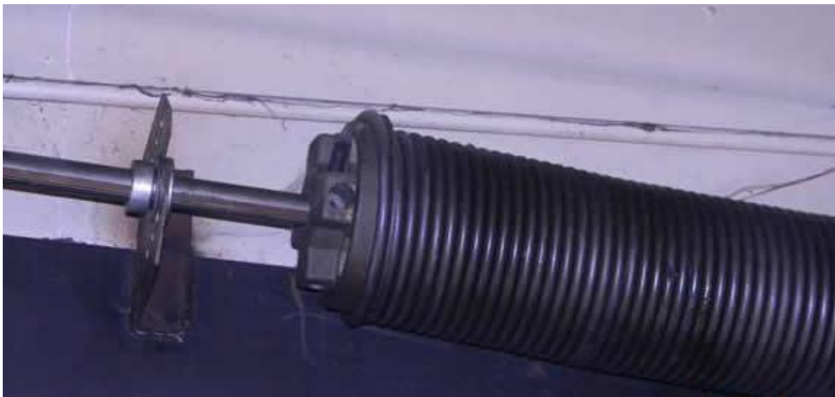
Figure 1: Overhead door springs are a dangerous source of stored energy.
