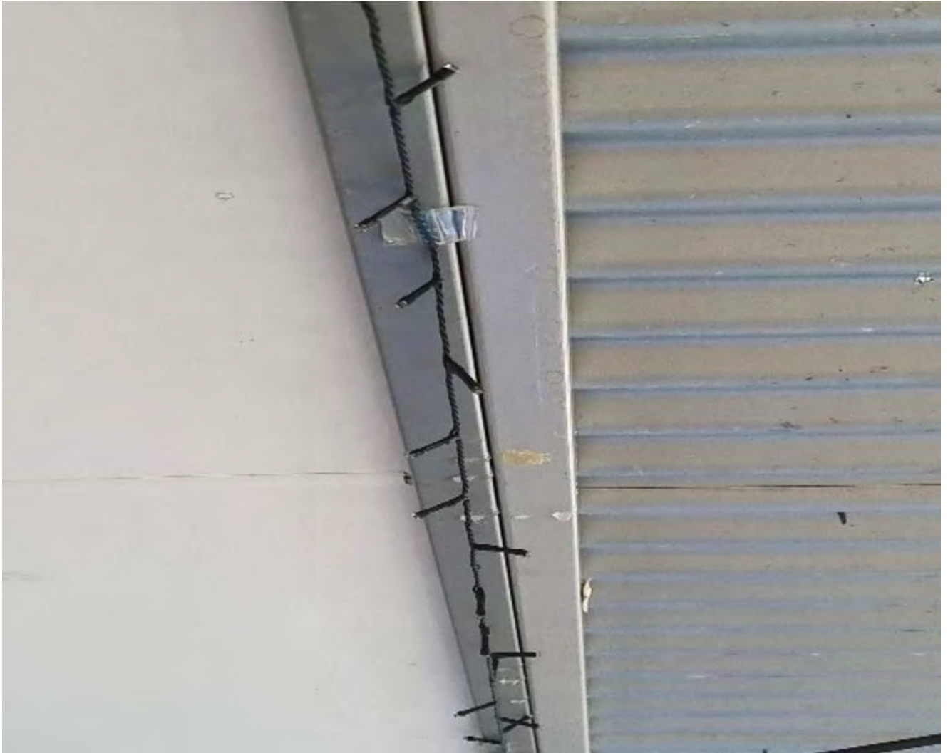
Figure 3. Patio join to main building
