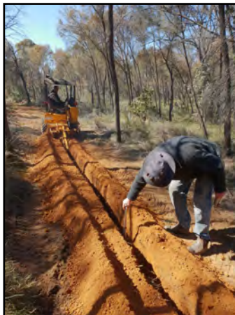
Graydn checking the depth of the trench.
