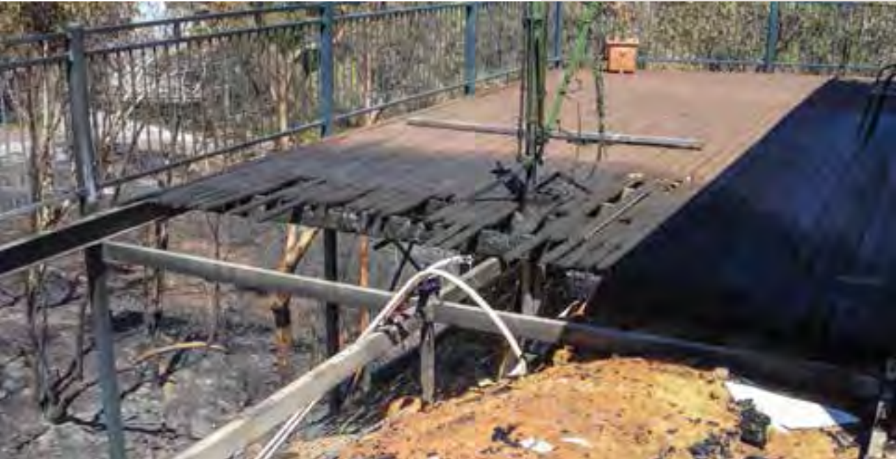
Below: Deck damage as a consequence of being constructed from inappropriate materials for the potential BAL.
