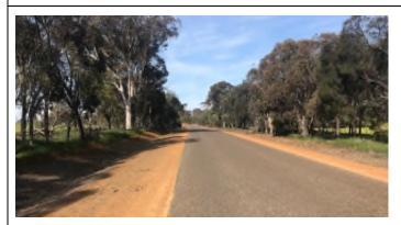
Road seal edge and shoulders are in good condition. Minimal signs of drop off or edge damage.
