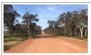
Gravel road condition shows good crown and drainage. This is a good technique for controlling depreciation of the asset.
