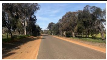
Roadside drains are free of large trees, and debris. There was signs of a weed spraying program in the rural drainages. This is a very good practice to maintain drains efficiently.
