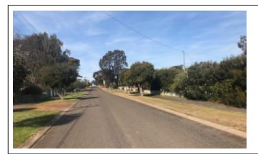
Seal and kerbed roads are in good condition. There is no signs of missing aggregate of erosions against the kerb face.
