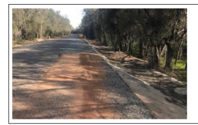
A recent pavement repair was inspected. It was found that the poor/failed pavement material was removed and replaced with suitable gravel material. This is a very good practice, and contributes reducing asset deprecation.
